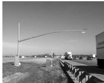
Participating PrePass trucks are checked by driving past sensors at highway speeds that verify compliance with state weight, safety, and credential requirements.
